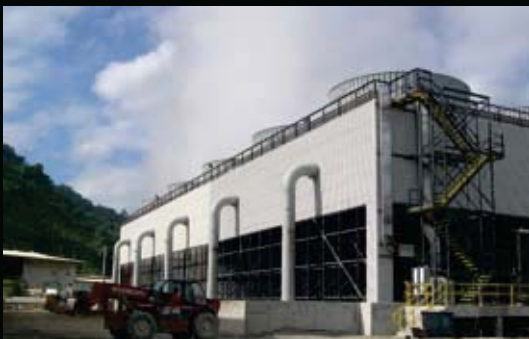
10-Cell Counterflow Tower - Geothermal - New Guinea
